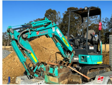
Figure 16. A Kobelco excavator used in the Byford rail extension project.
